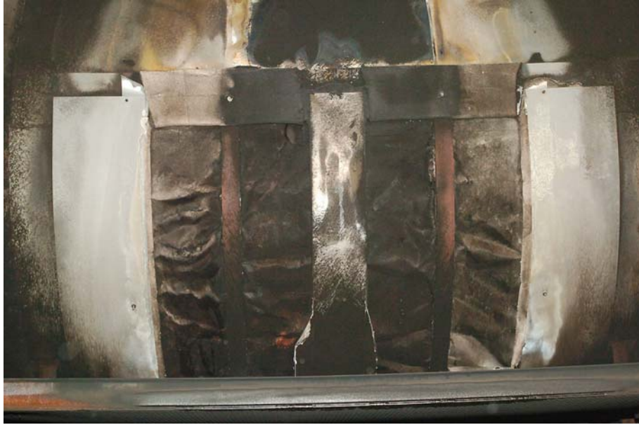
Figure 51. Posttest Inspection of the Fiberglass/Ceramic Barrier Insulation System
