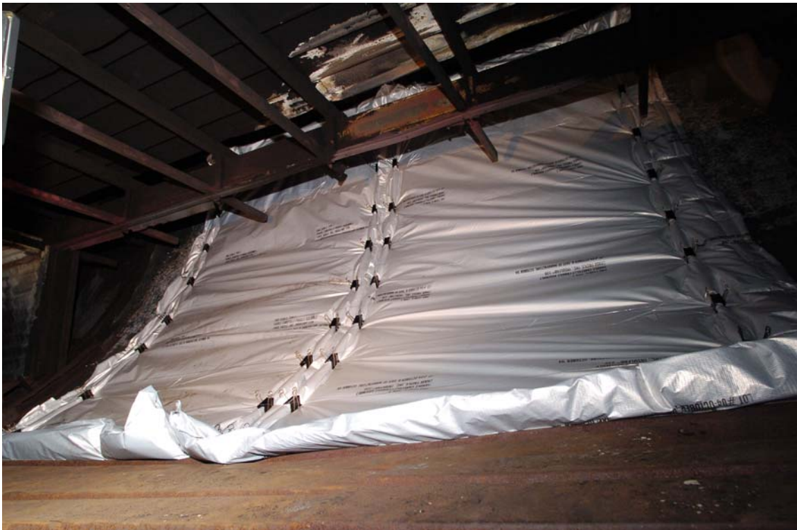
Figure 48. Installation of Blankets Containing the Thin, Ceramic Barrier and Fiberglass Insulation
