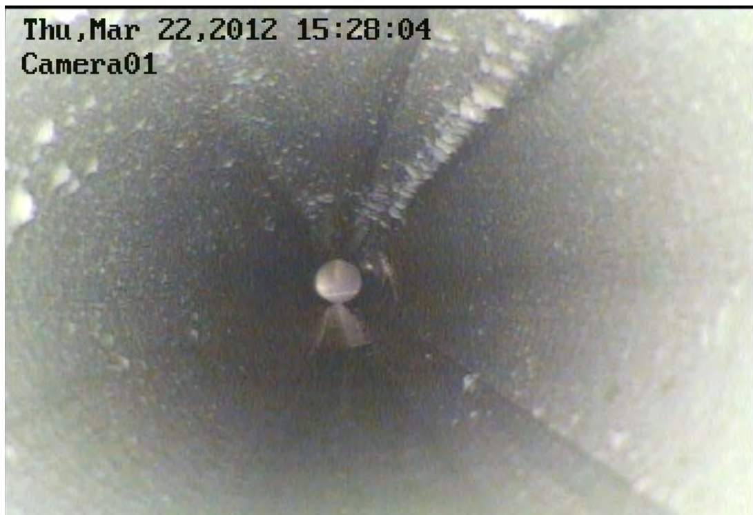
(b) Downstream Pipe Section
