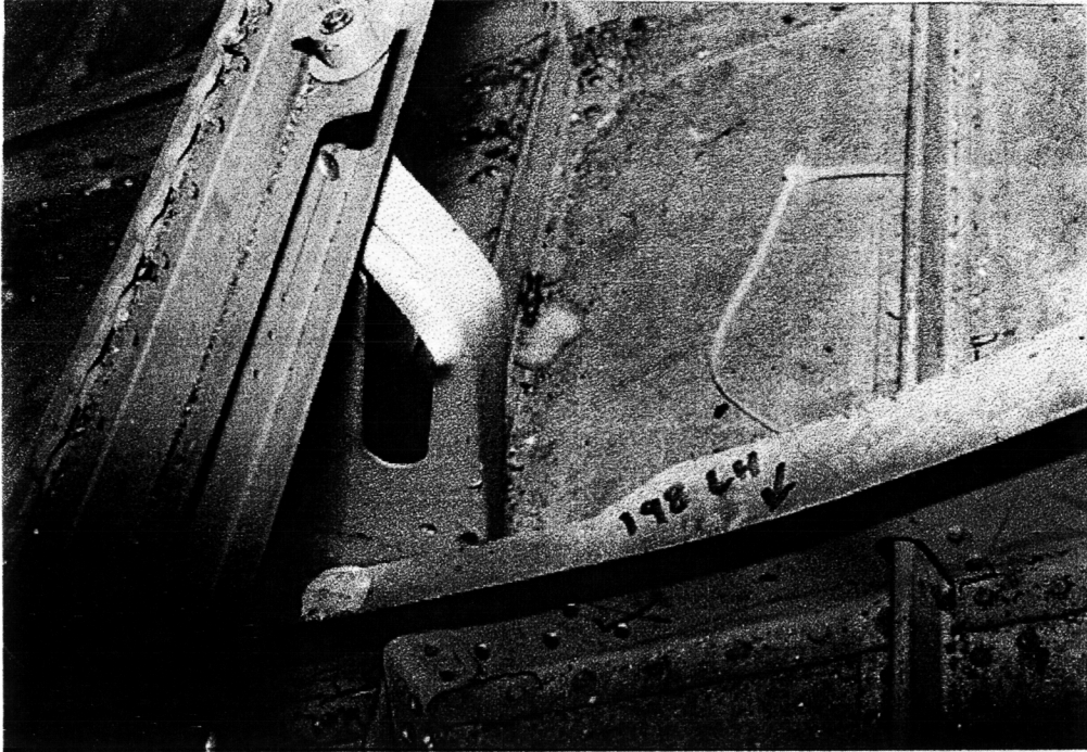
FIGURE 20. UNDERFLOOR BUCKLING L/H SIDE, AFTER IMPACT
