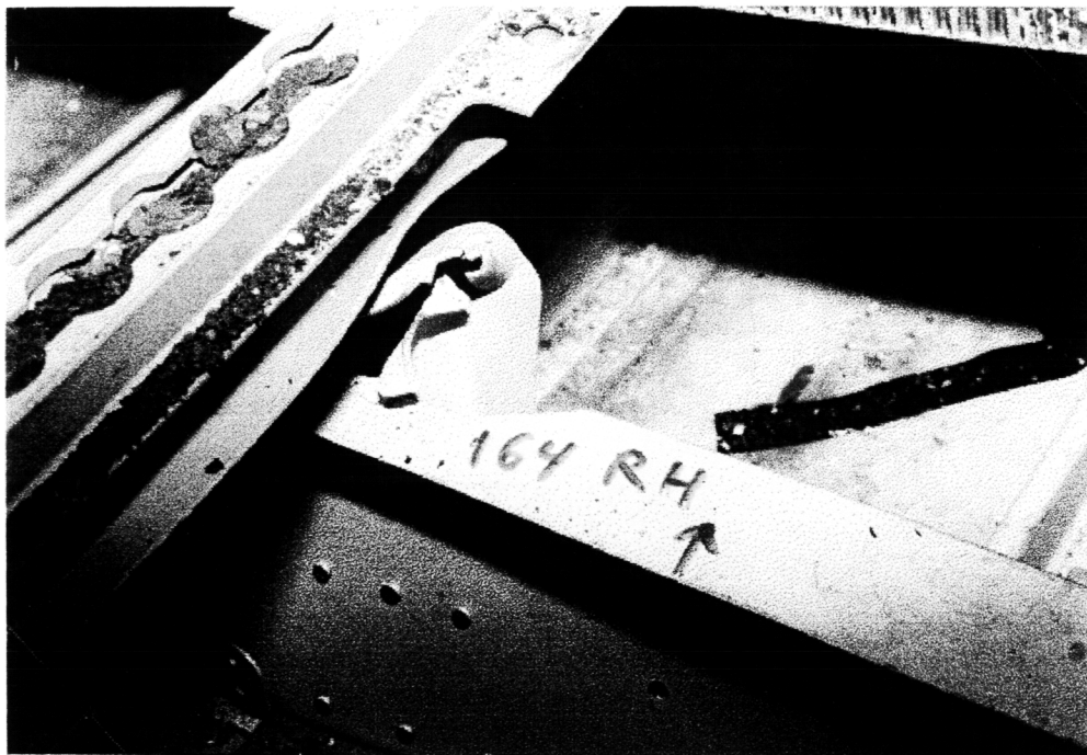
FIGURE 19. UNDERFLOOR BUCKLING R/H SIDE, AFTER IMPACT
