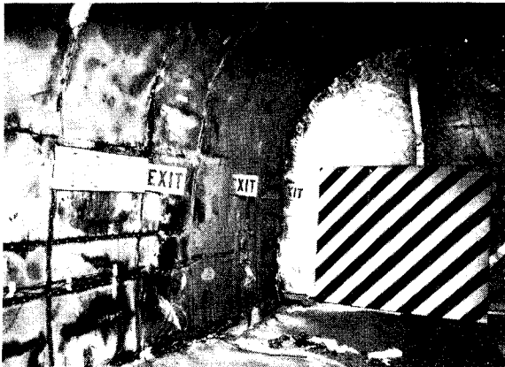
Interior of protected section after test. South side.
