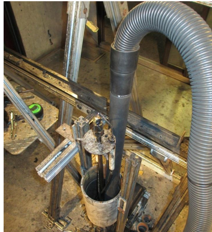
Removing soot with vacuum
