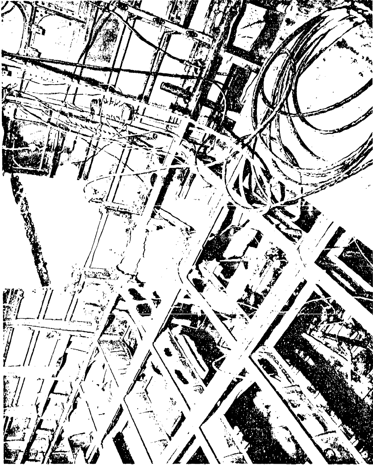
FIG. 2.4 INTERIOR STRUCTURAL DAMAGE AFTER TEST NO. 4
