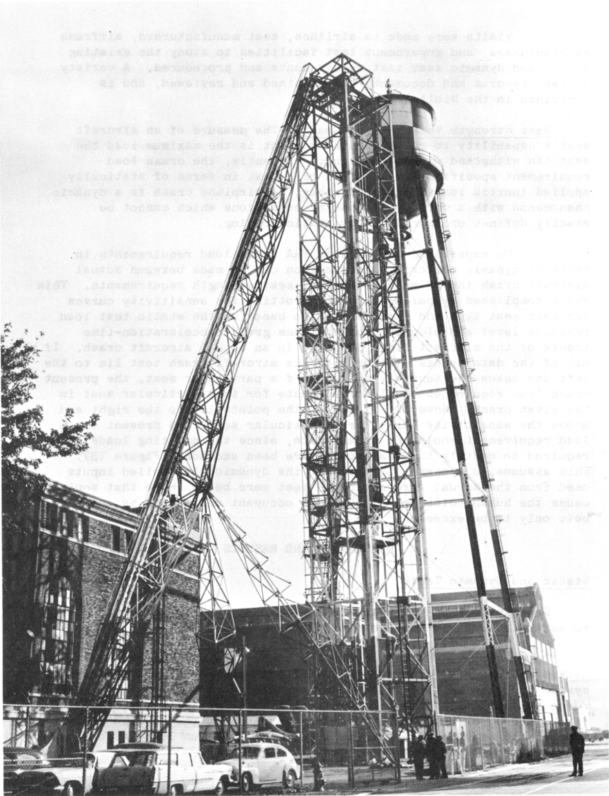
FIG. 12 ACED 150-FOOT VERTICAL DROP TOWER
