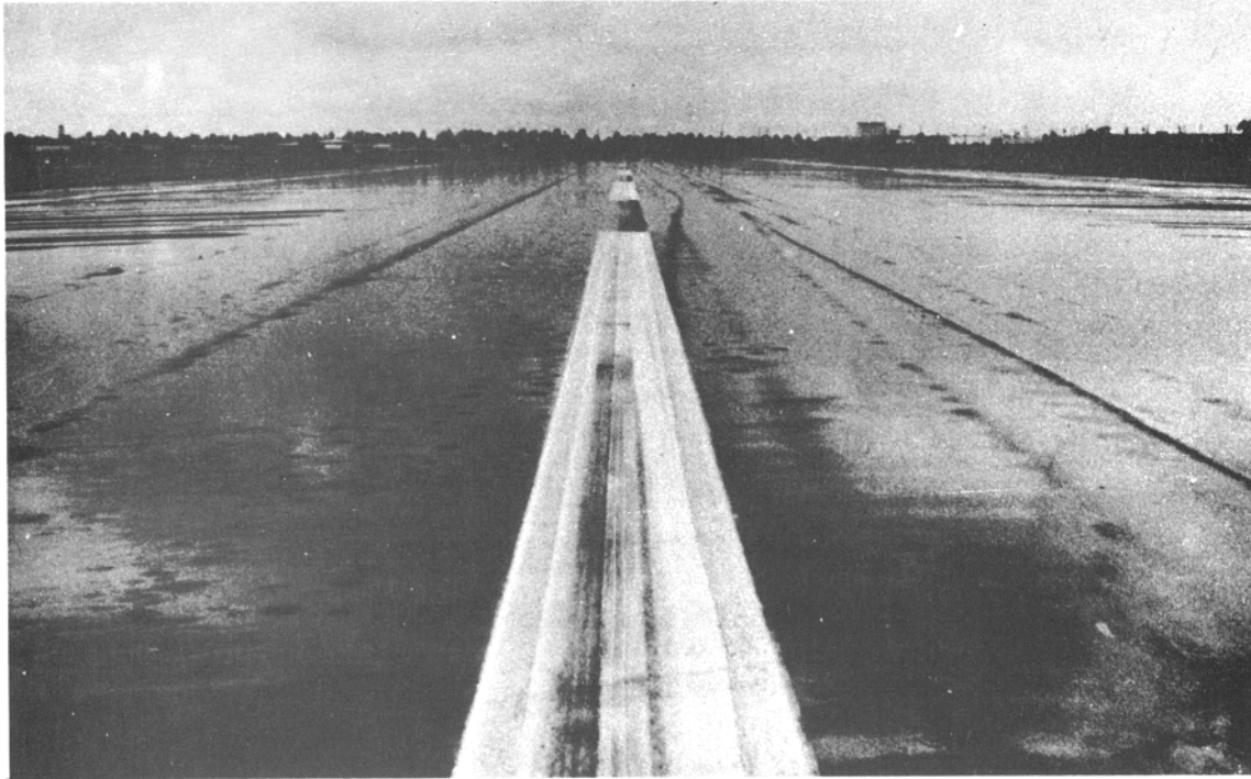
FIGURE 11. RUNWAY WETNESS AFTER A MAXIMUM WET TEST HAD BEEN COMPLETED
