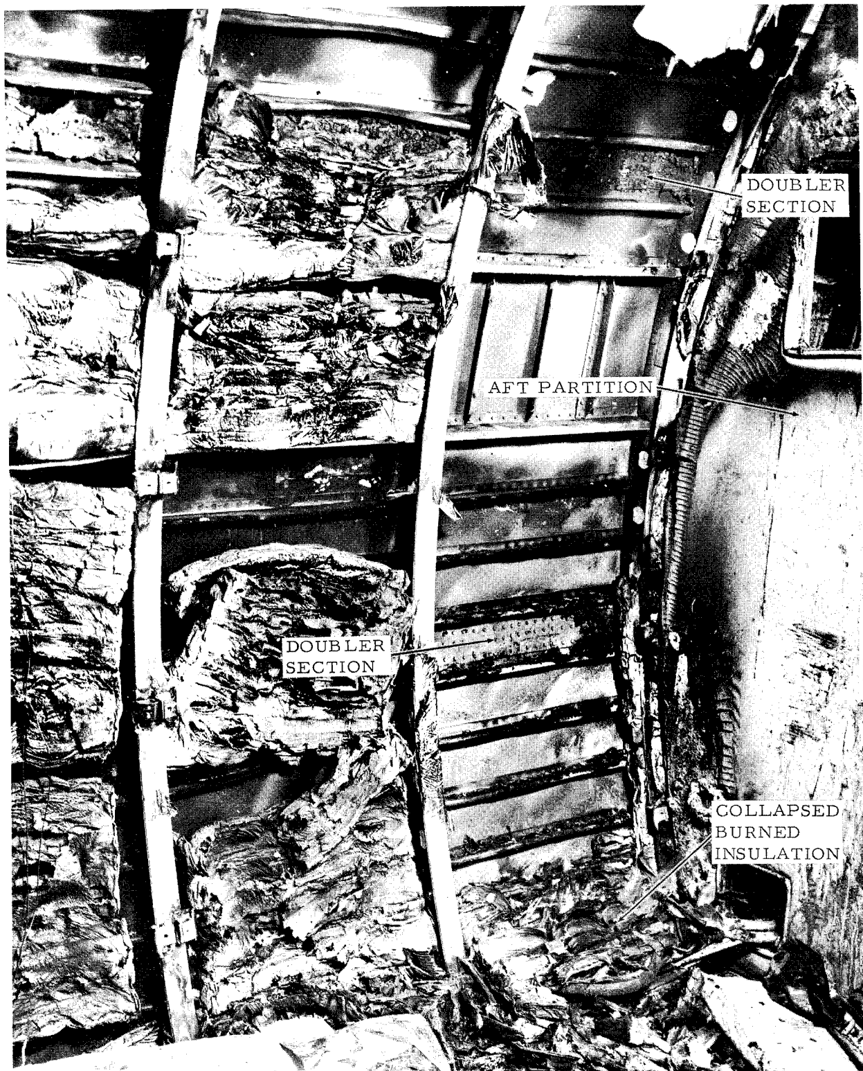
FIGURE 17 - BURNED SEALANT AND INSULATION NEAR AFT END
