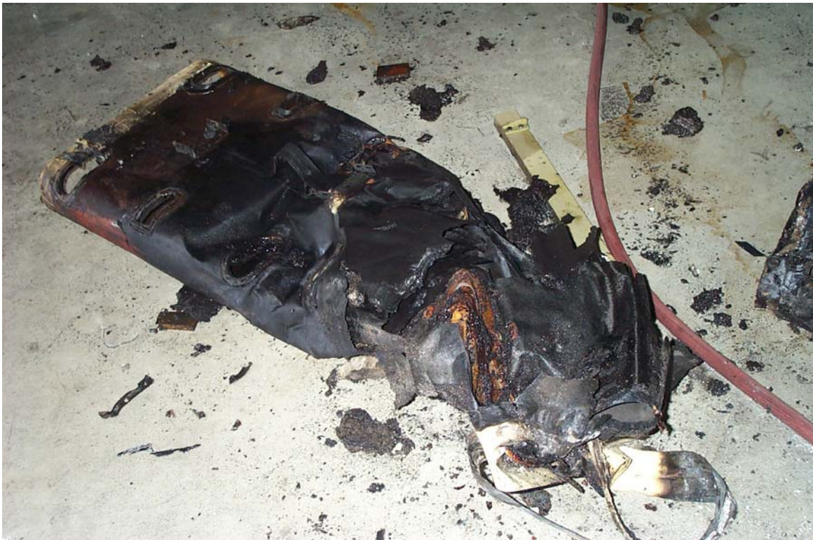
FIGURE 13. POSTTEST CONDITION OF AIR CONDITIONING DUCT
